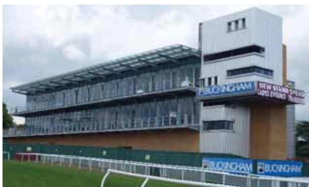
Advanced progress on the construction of Fontwell's new Premier Grandstand, due to open in August 2010, aided by a £4m loan from the Board's Capital Fund in 2008/09.
